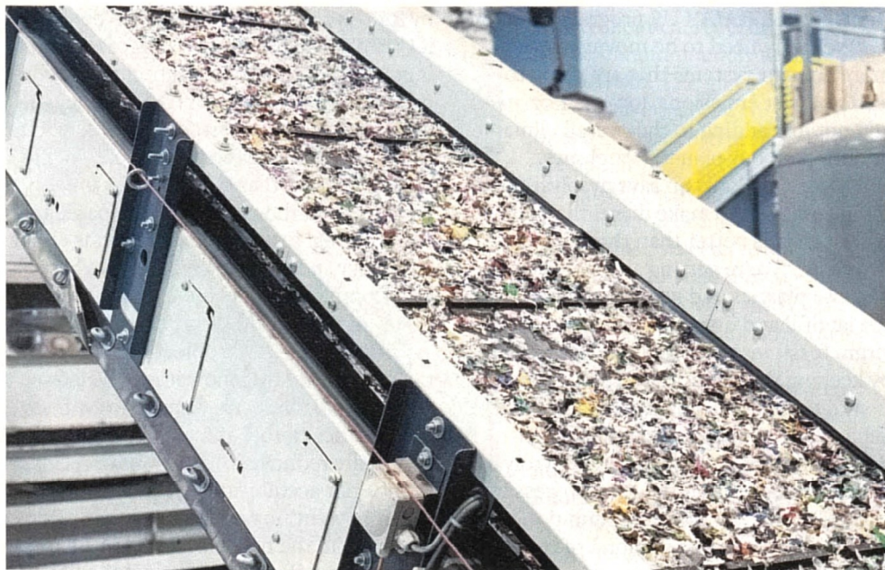
Brightmark is testing equipment at its plastics pyrolysis plant in Ashley, Indiana.
