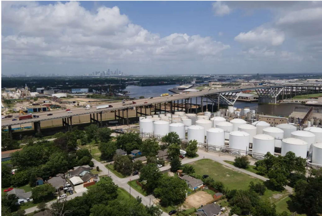
An overhead view of the Valero refinery on May 12, 2023 in Houston. Credit: Mark Felix, Grist
